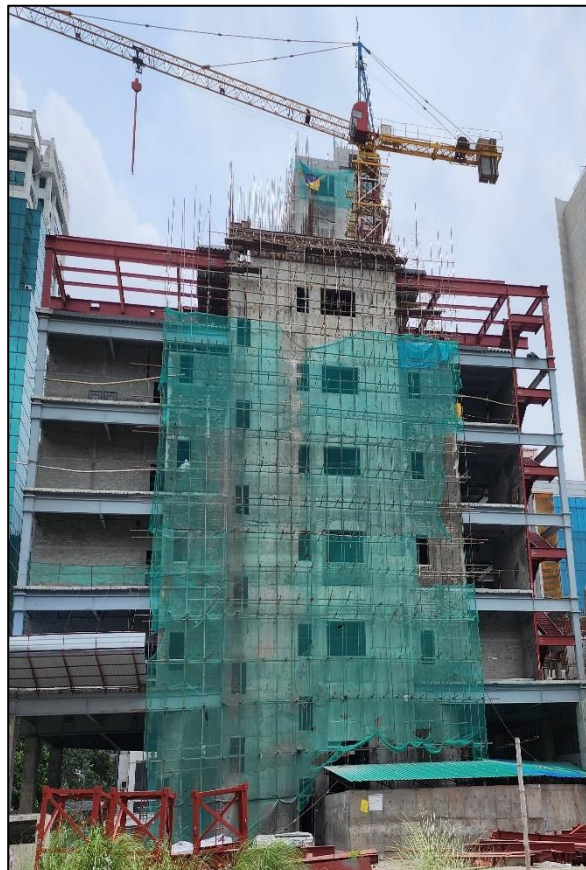
Under construction URU building
