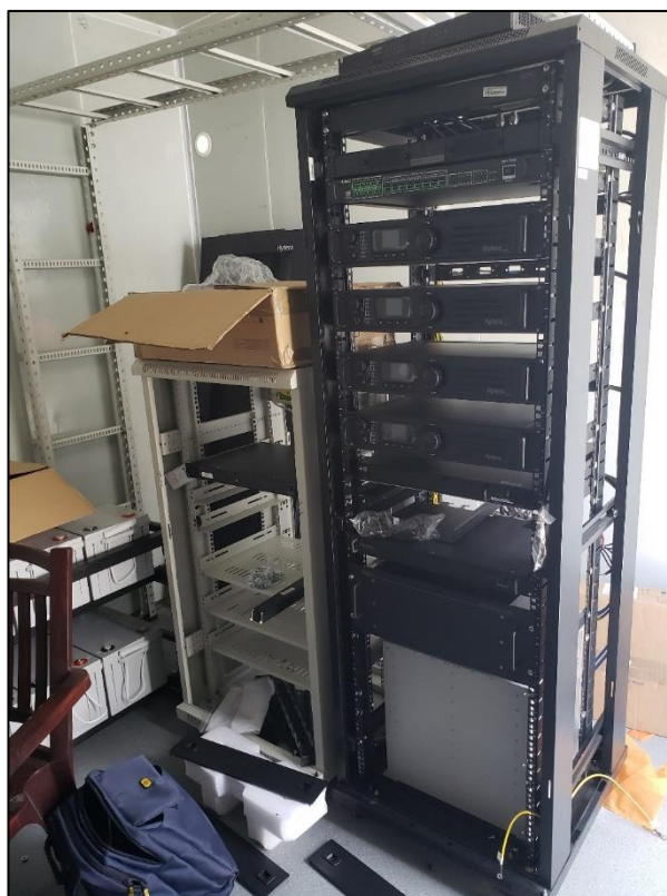
Installation of DMR Network at Rooftop base station
