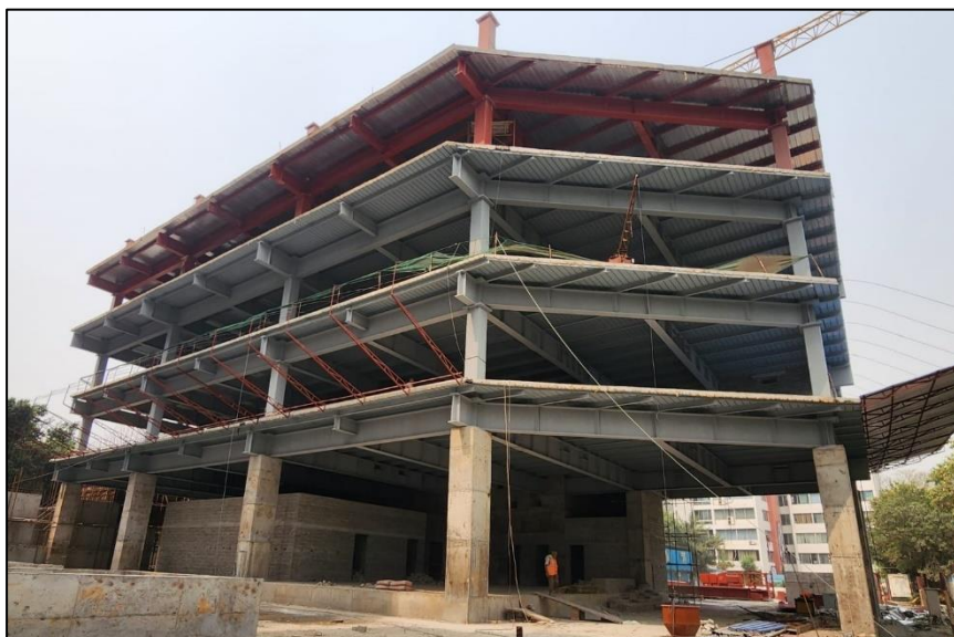
Ongoing construction of Urban Resilience Unit (URU), RAJUK
