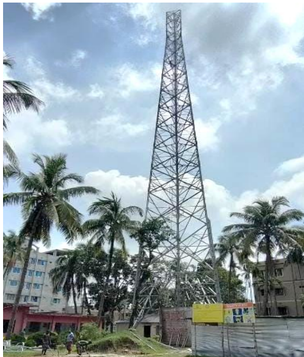
Ongoing work of Green Field tower
