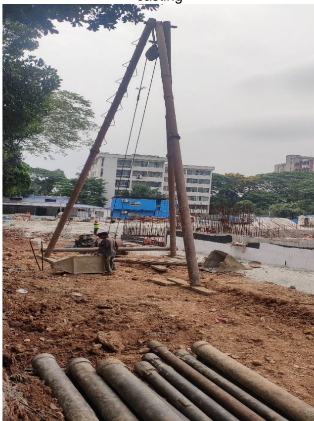
Piling work is going on for laboratory building
