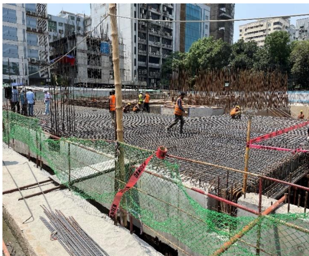
Preparation for floor (B1), ramp, and lift core casting
