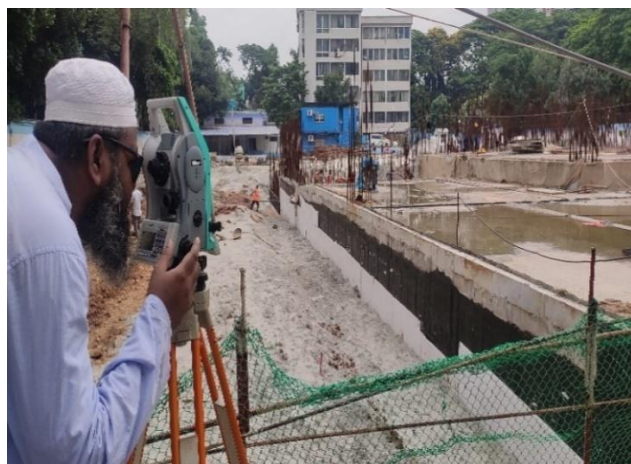
Level checking work is on-going
