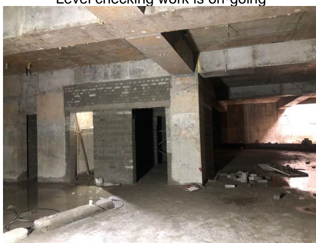
Lobby area of Basement-1
