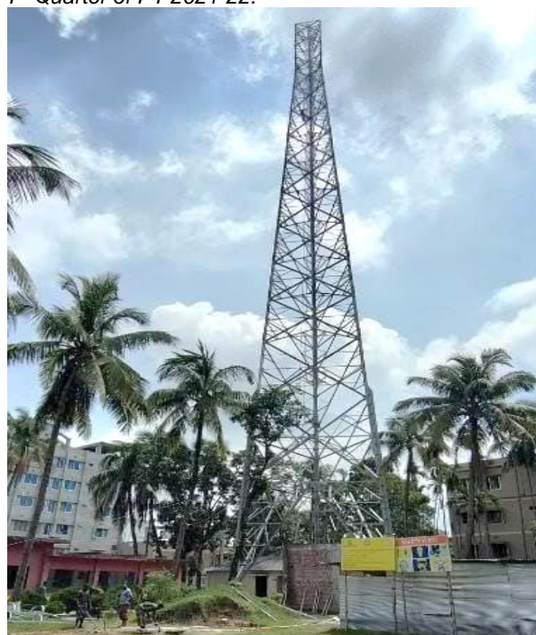
Ongoing construction of Green Field tower
