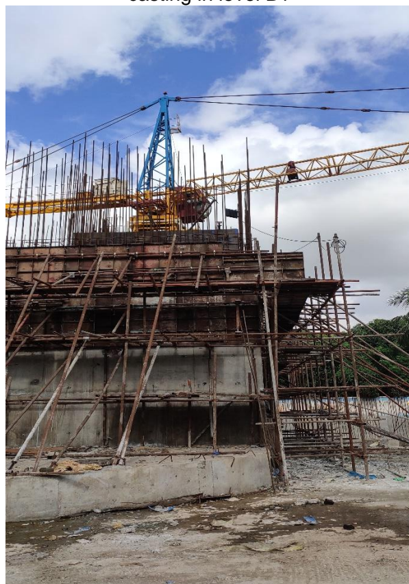
Tower crane fixing work is on-going
