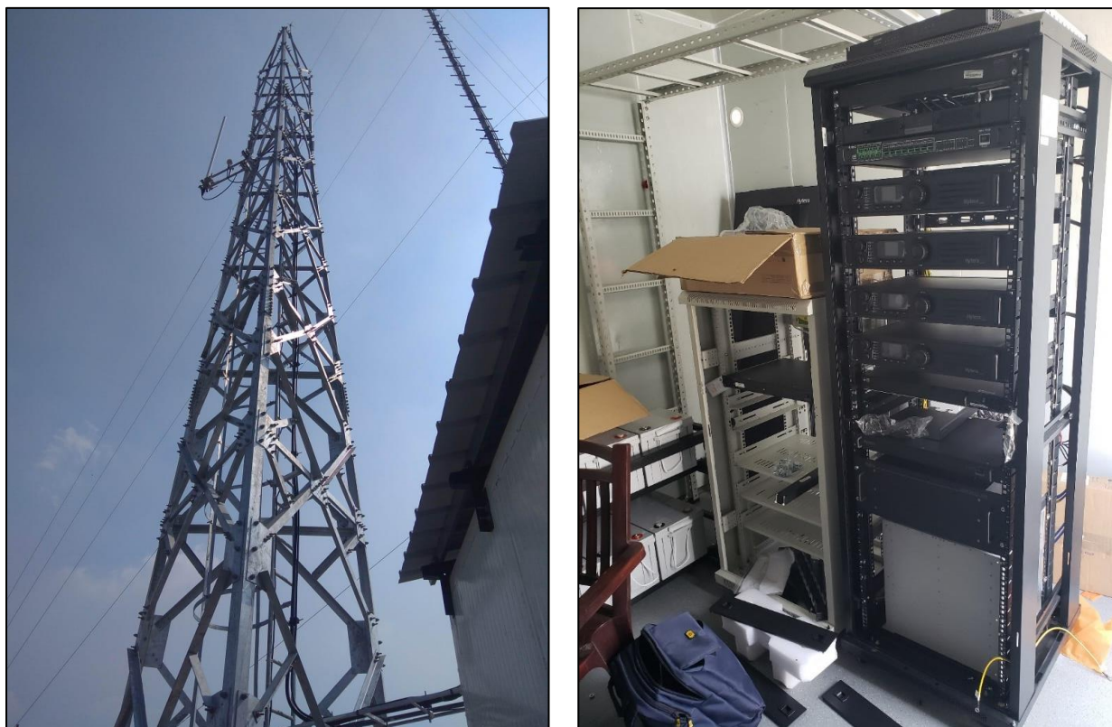
Installation of DMR Network at Rooftop base station
