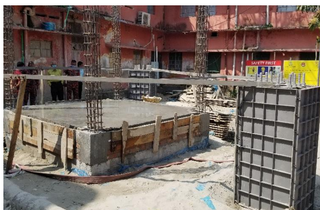
Ongoing Column casting work of Green Field tower
