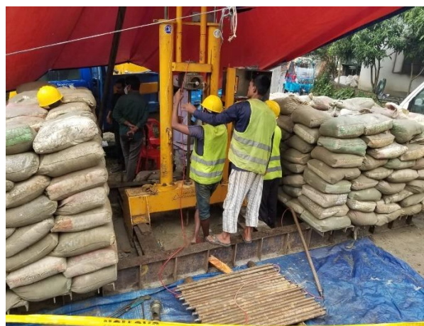
SCPT field survey on-going at Keraniganj site of Dhaka (December 5, 2021)
