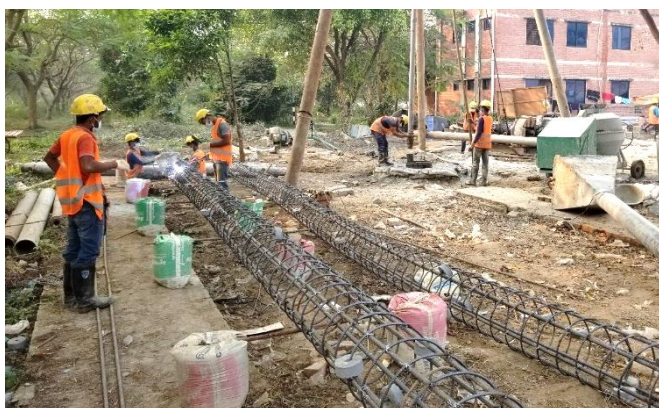
Ongoing pile reinforcement work of Green Field tower
