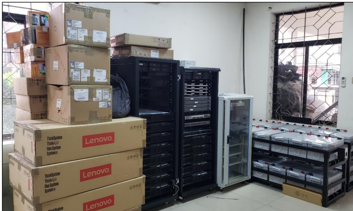
Digital Mobile Radia (DMR) Network at FSCD
