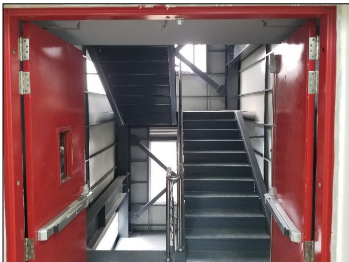
Constructed Emergency Exit
