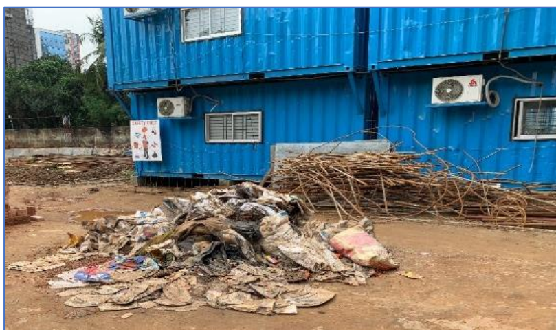
Wet, contaminated rags, scraps, lying. June' 21
