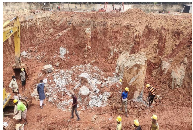
Earth work excavation
