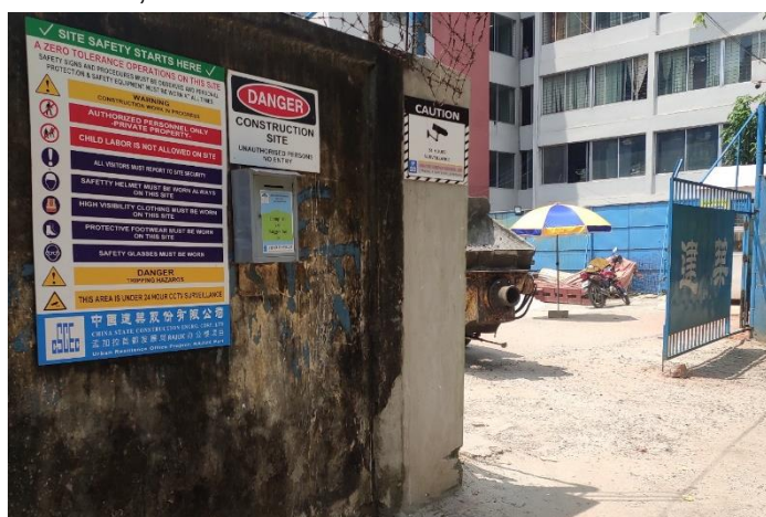
Installation of Complaints and Suggestion box in a visible area
