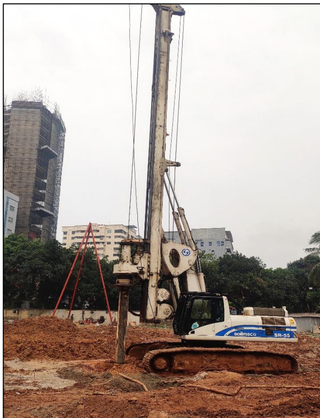
Borring work by hydraulic drilling rig
