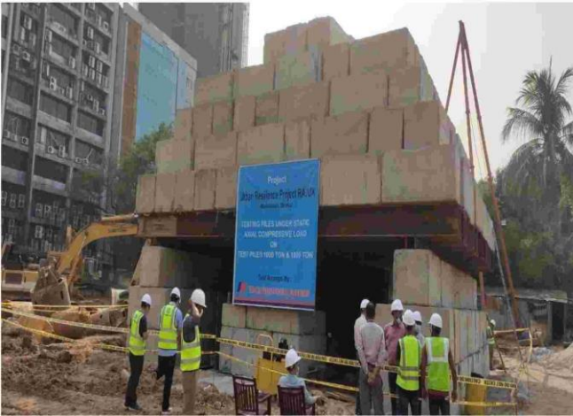
Static load tests for service piles
