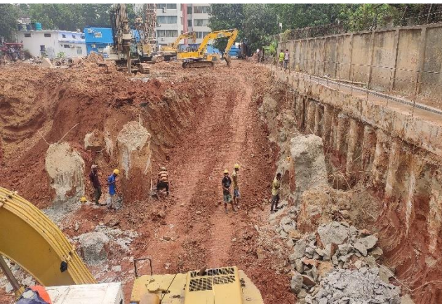
Earth work excavation
