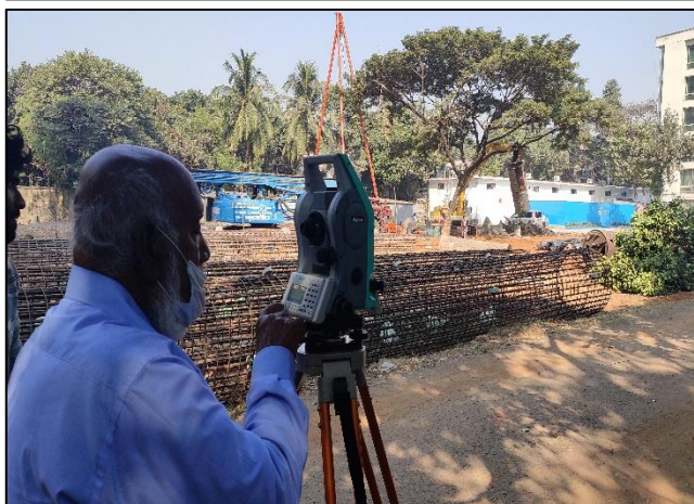
Re-bar binding works
