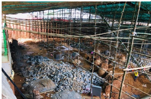
Construction of rain-water shed
