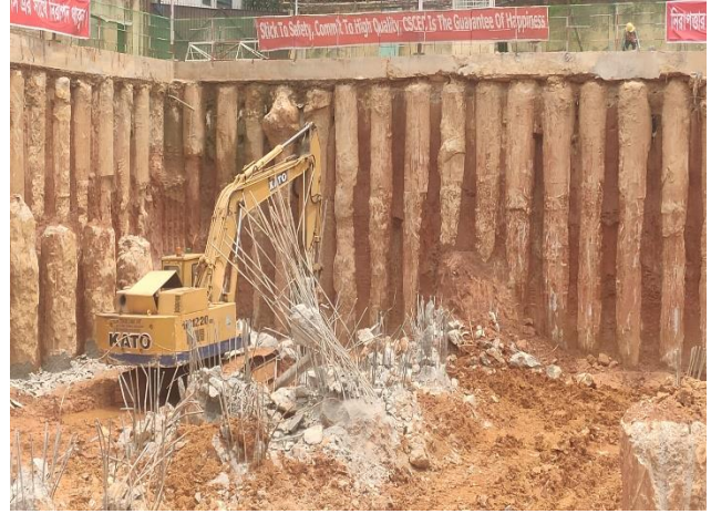
Earth work excavation
