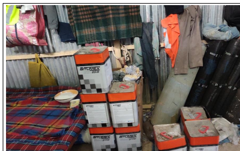
Risky storage of bitumen inside the worker's camp
