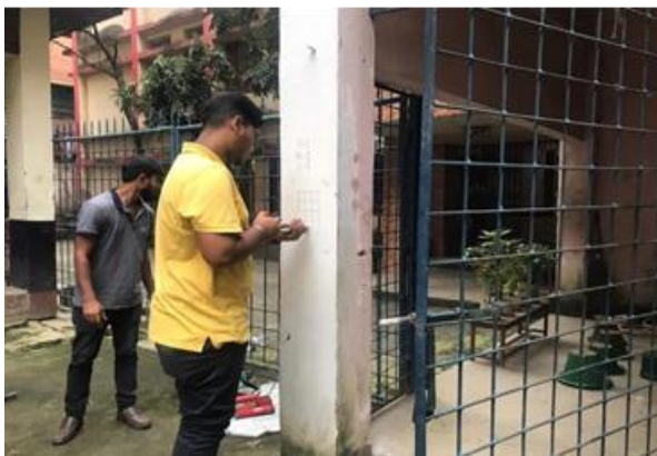
Re-bound hammer test
