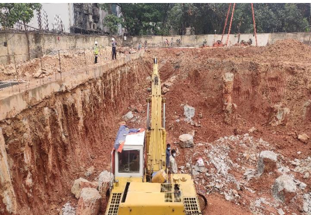
Earth work excavation
