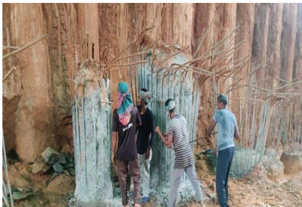
Pile-cap breaking work
