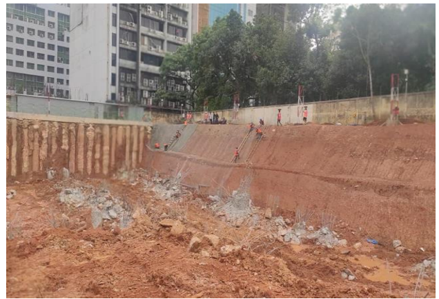
Side protection work by wire-mesh
