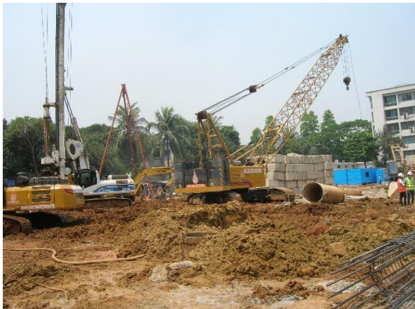
Unsafe drop-off without any warning signs or barriers to prevent falls or other injuries.
