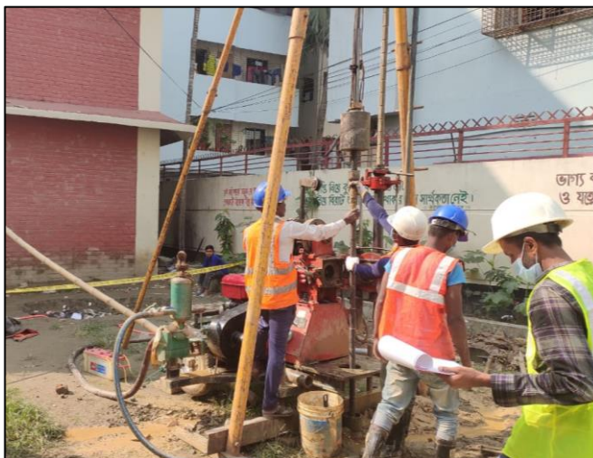
Ongoing Standard Penetration Test (SPT)
