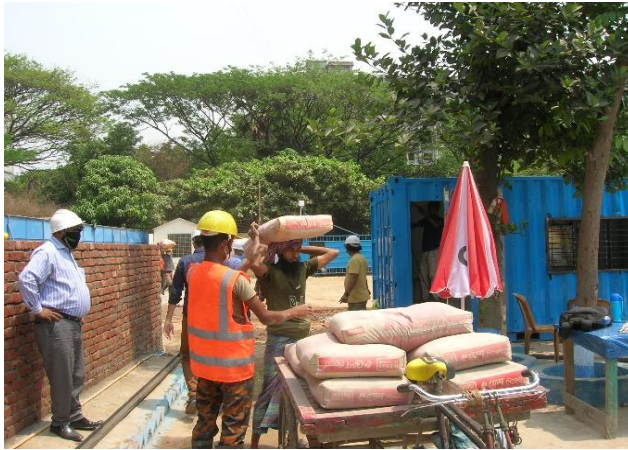
Workers without helmets, eye and ear protection, or N95 masks to reduce inhaling hazardous airborne particulate matter (cement dust in this case).
