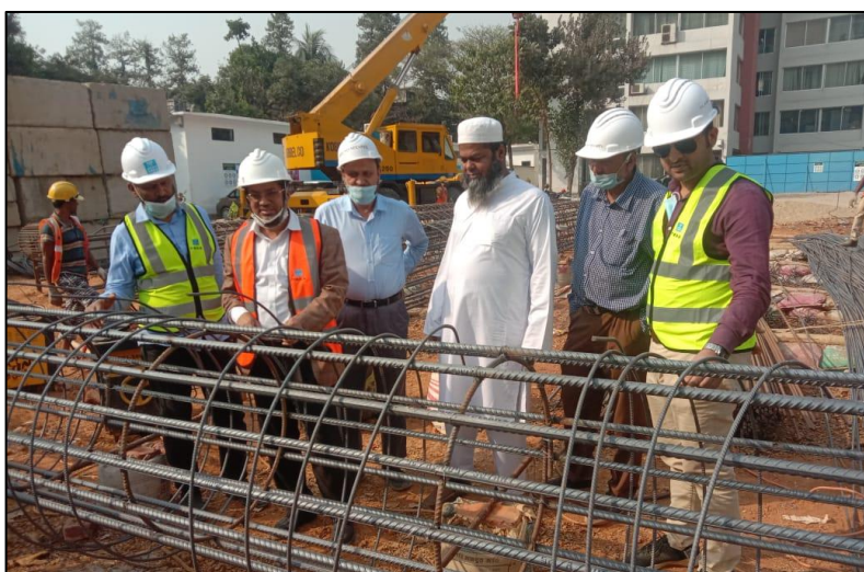
Field Visit to URU Construction site
