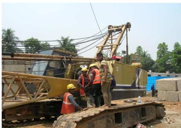
Lack of personal protective equipment amplifies employee's exposure to hazards, increasing risks.
