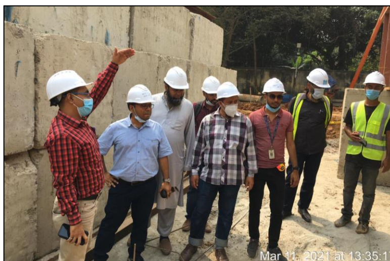
Field visit to monitor load test arrangement
