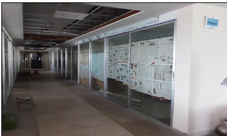
On-going ERCC Renovation Work
