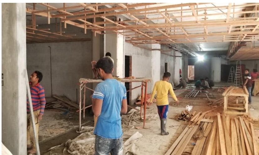
On going Construction of EOC in DNCC, Nagar Bhaban, Dhaka.
