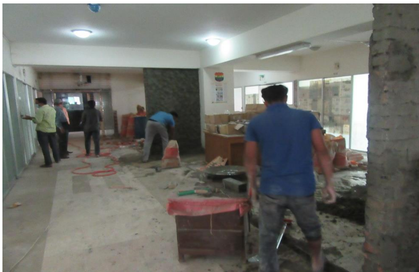
NDMRTI Renovation work on-going
