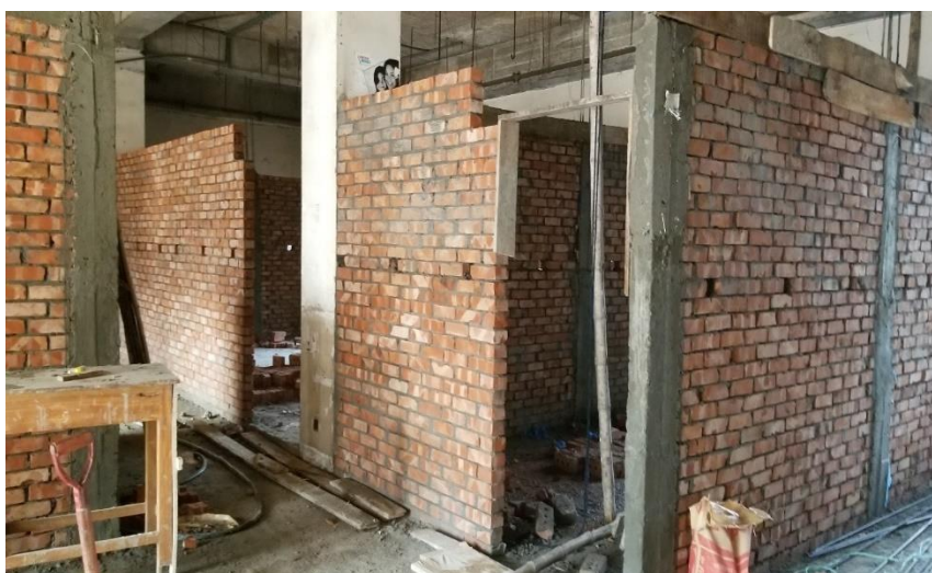
On going Construction of EOC in DSCC, Nagar Bhaban Dhaka.
