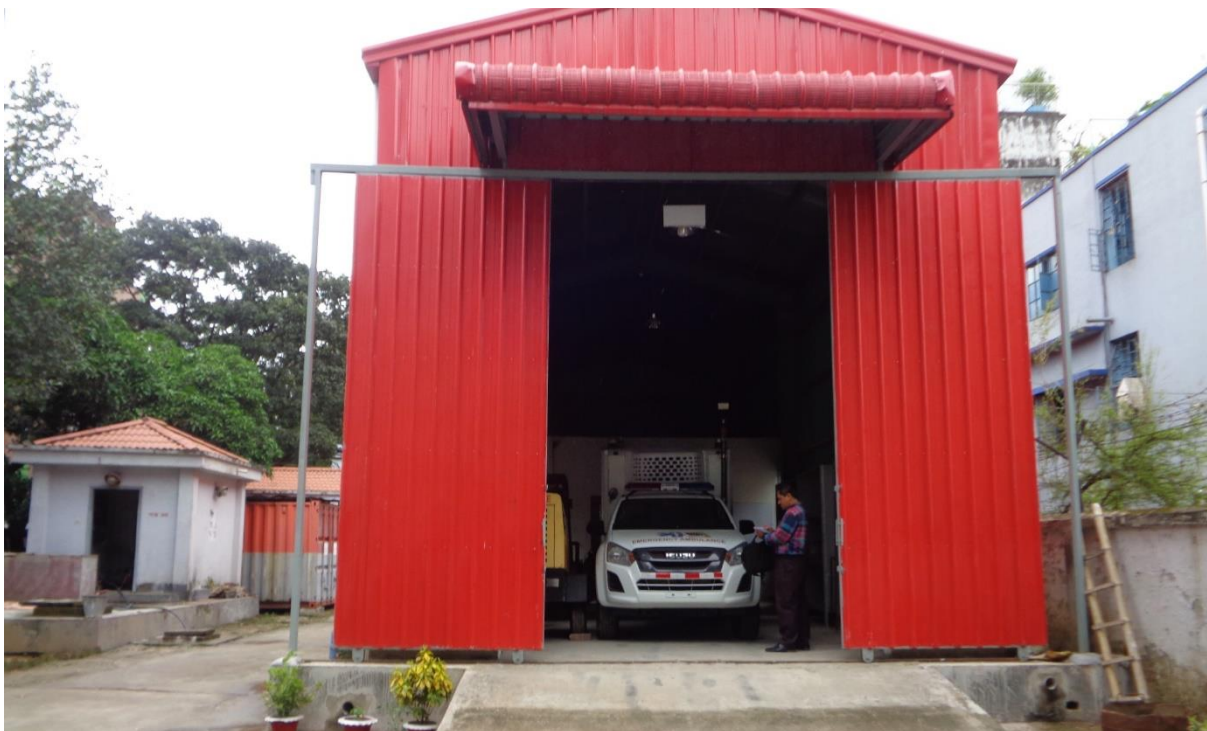
Figure 6: FSCD Warehouse, Khilgaon
