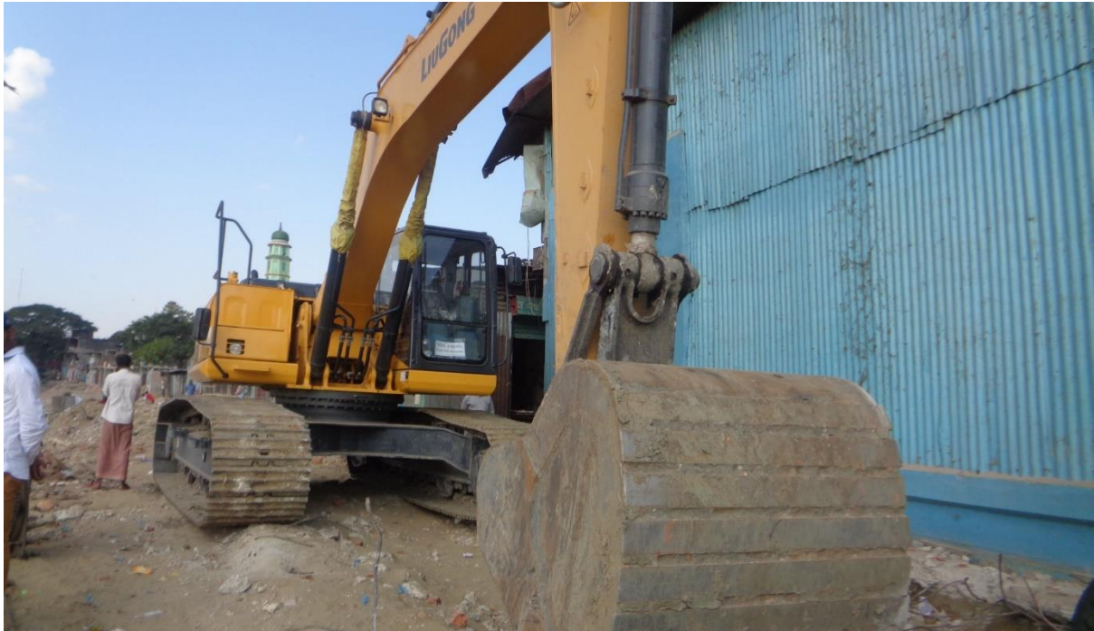
Figure 17: Chain Type Excavator for DSCC, DNCC & SCC (3)
