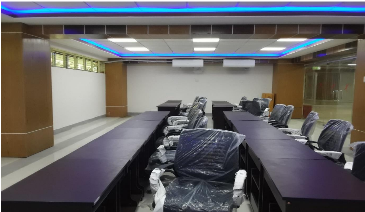
Figure 18: Renovation work of ERCC of DDM
