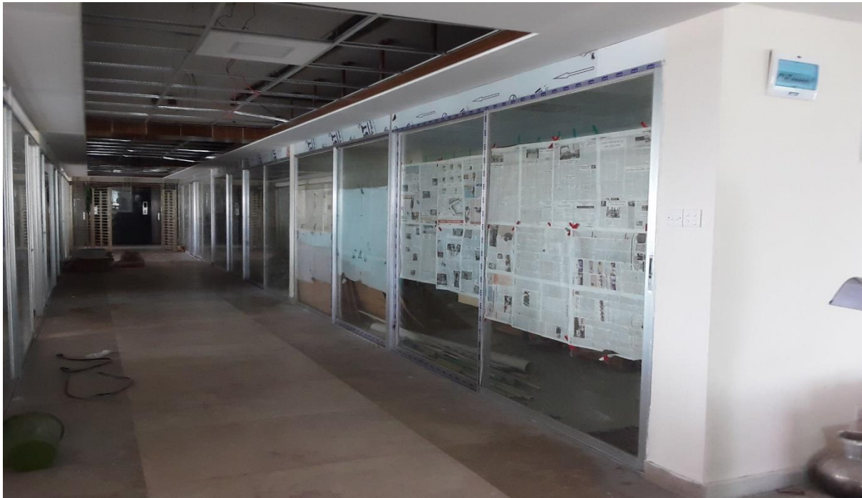
Figure 19: Renovation work of ERCC of NDMRTI
