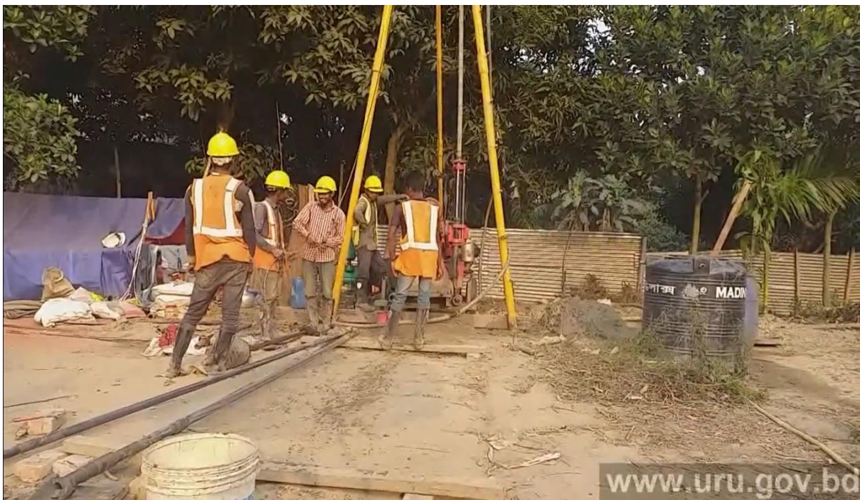
Figure 24: Standard Penetration Test (SPT); RAJUK
