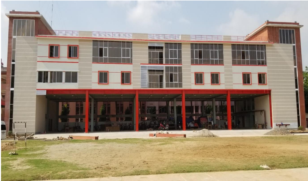
Figure 1: Command and Control Center with Warehouse of FSCD Training Academy, Mirpur-10
