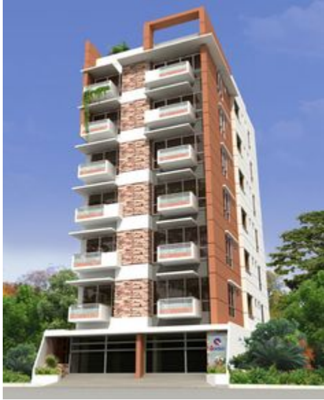
Figure 8-28: Two random examples of soft-story buildings
