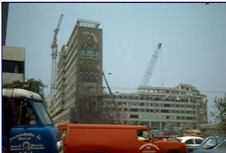
Figure 8-26: The Ministry of Transportation and Telecommunication building following the Mexico earthquake of 1985
