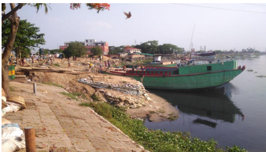
Figure 2.19 An embankment in the western part of Dhaka
