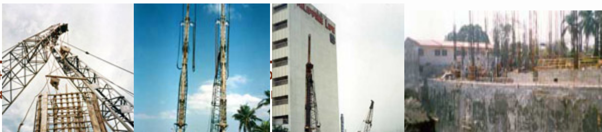
Diaphragm wall rigs
