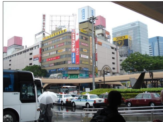
Post-earthquake view of downtown Sendai, located only 130 km from the epicenter of the March 2011 Tohoku earthquake, where one had to look for damage, which occurred predominantly in the older buildings.
