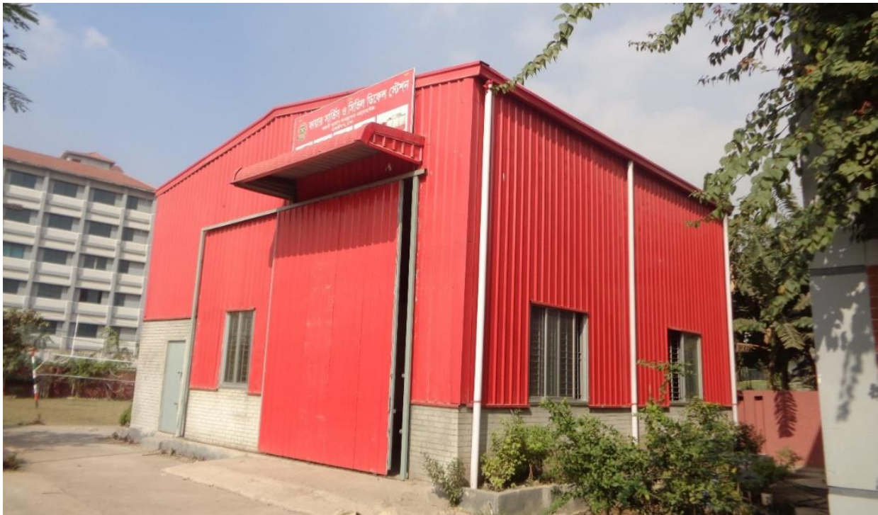
Figure 6: Constructed Warehouse of FSCD in Hazaribag
