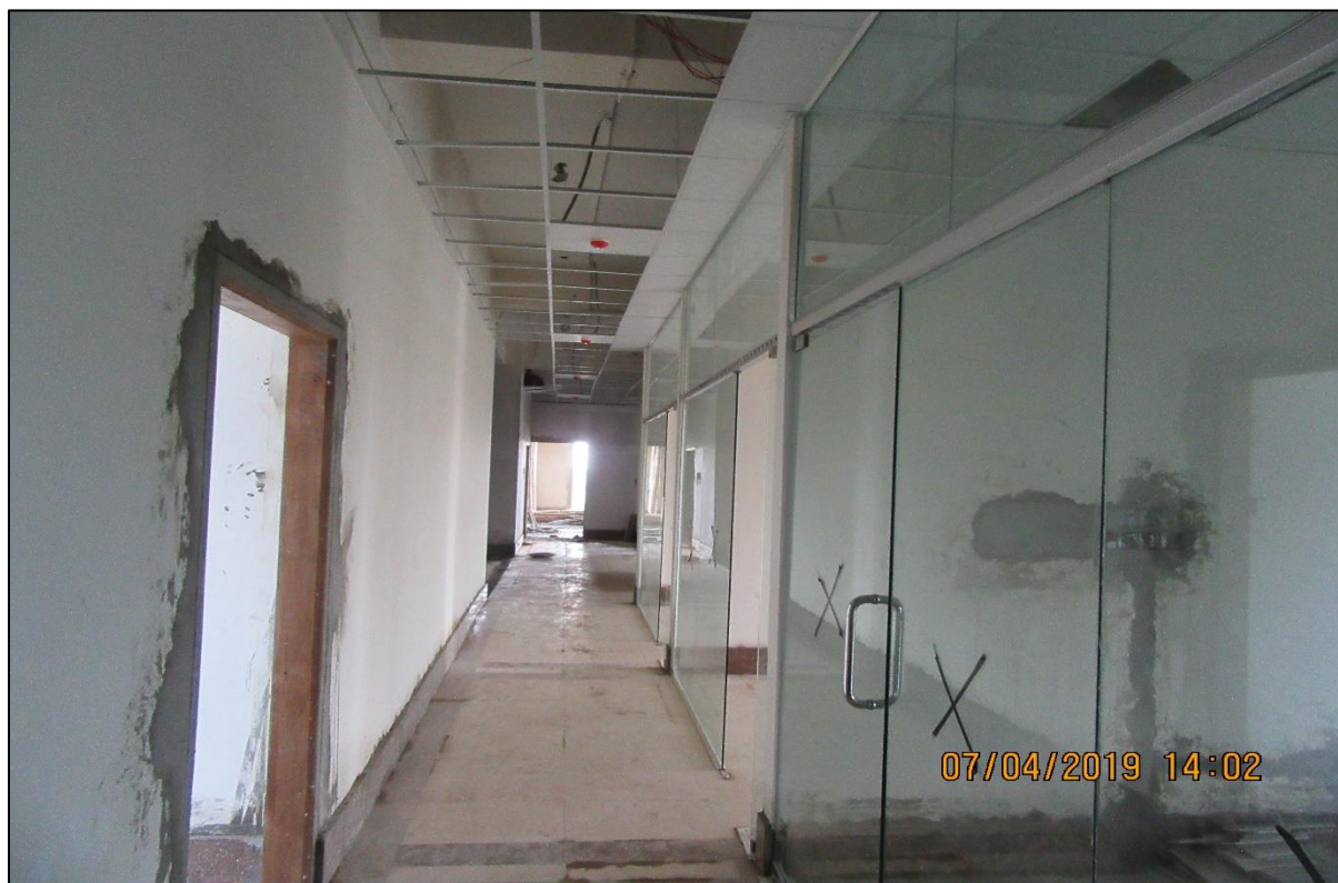
Figure 3: Construction of EOC in 5 th floor of Nagar Bhaban, Sylhet.
