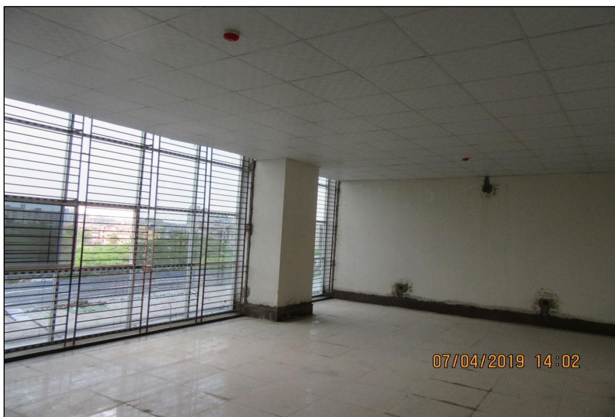
Figure 4: Construction of EOC in 5 th floor of Nagar Bhaban, Sylhet.
