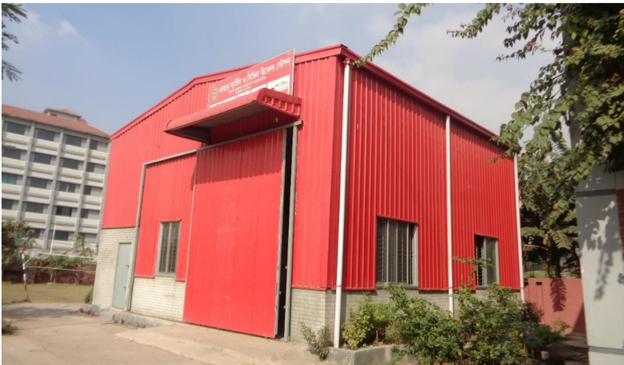
Figure 4: Constructed Warehouse of FSCD in Hazaribag
