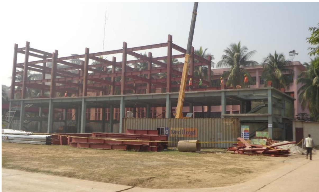
Figure 6: Constructed Warehouse and Command & Control Center of FSCD in Mirpur-10
